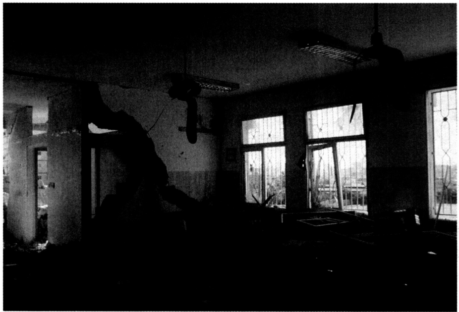
A classroom in the Al-Arqam elementary school, Gaza. The school was one of numerous targets bombed by Israel during "Operation First Rain" in October. See Elmer, "Air Raids Terrorize Gaza Residents, Target Key Infrastructure," The New Standard <newstandardnews.net>.
